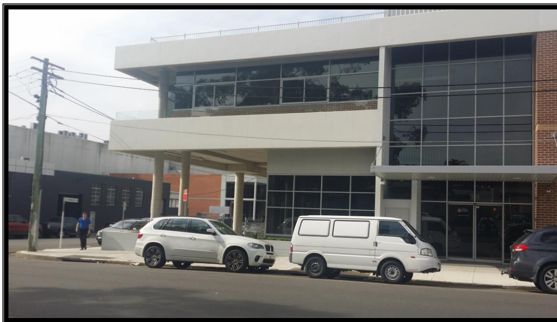
Photo 1: Site frontage to Regatta Rd at Spencer St
